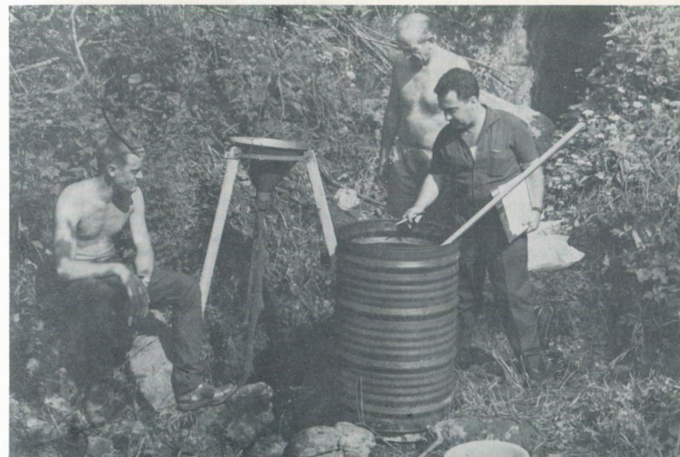
Figure 3. Scene at the swallow hole showing the barrel used to dilute the ammonium bromide and the funnel for introducing spores. Entrance to Feliefferhof cave in background, through which stream flows for a short distance.
